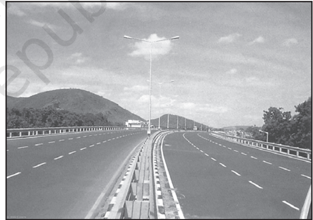
Fig. 7.3 : Dharmavaram Tuni National Highway, India
