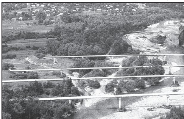
Fig. 7.17: Pipelines transporting natural gas in Ukraine
